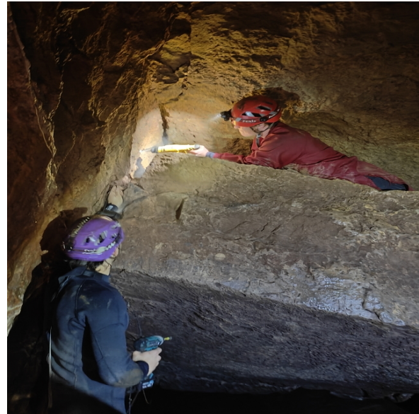
Scrubby Creek Cave installing the phone line
