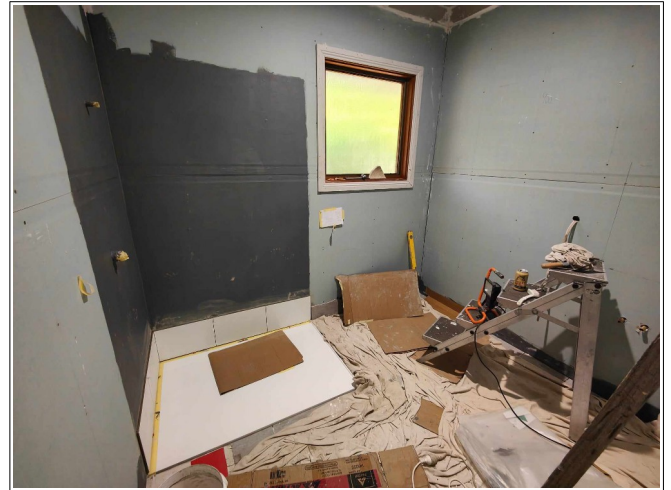
And the new bathroom with water-proofing and tiling activity under way.
