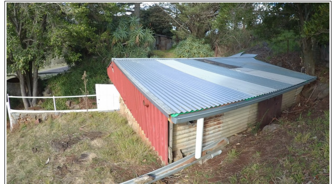
Showing off the new roofing over the cave entrance foyer
