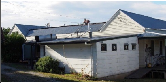
Homeleigh north wall and refurbished gables ( see larger photo )
