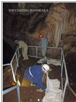
Hand rails painted ( see larger photo )
