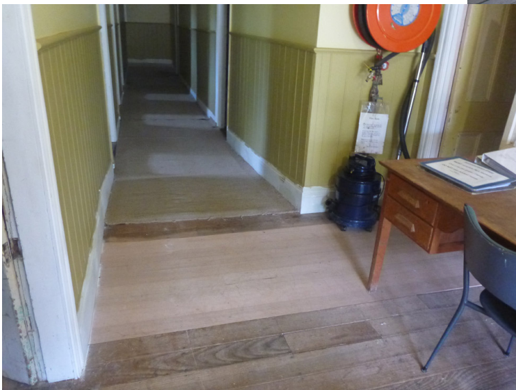
Repairs to the front hall floor
